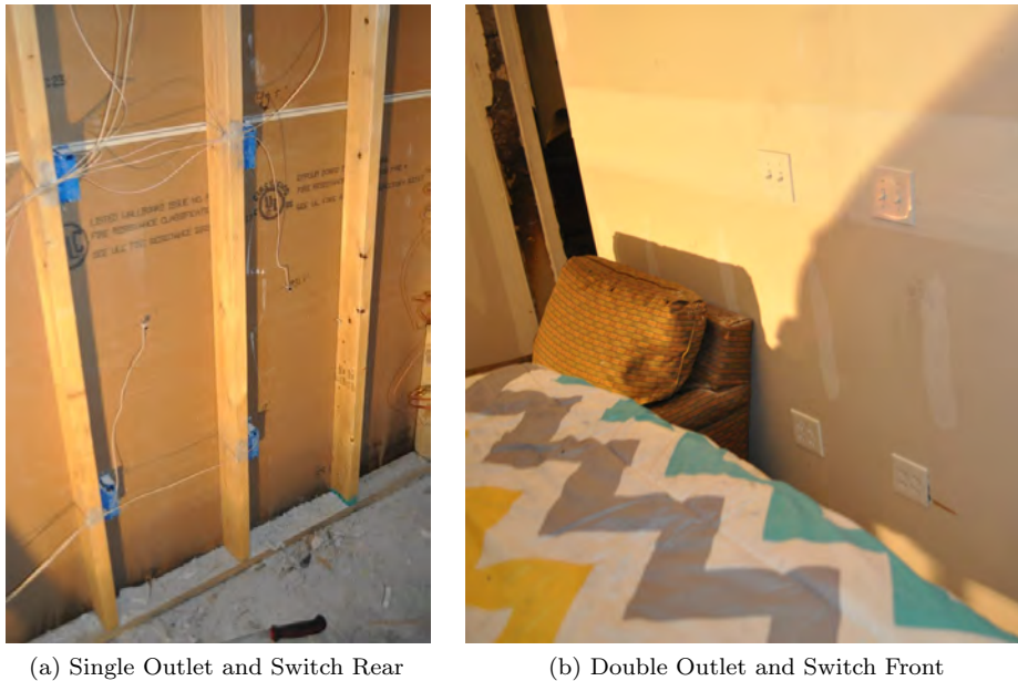
Figure 6.37: Void Space Wall Penetrations
