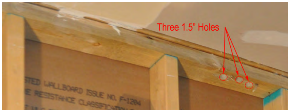
(c) Top Plate Configuration
