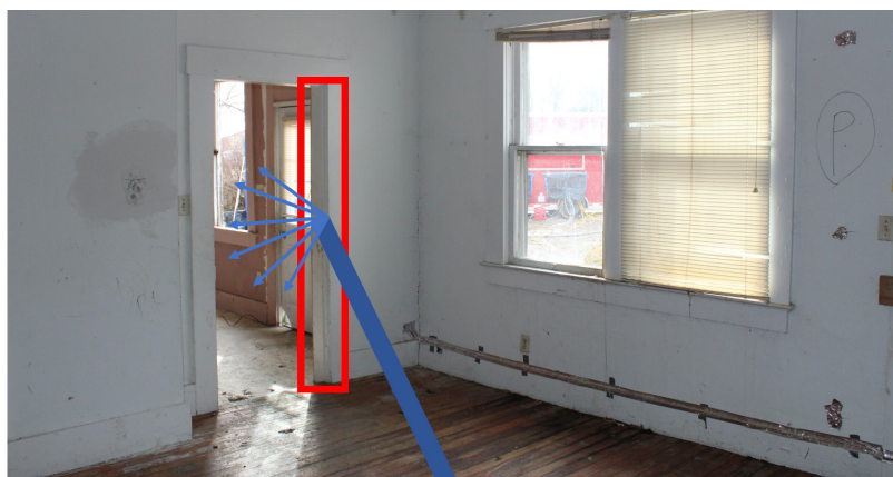
Figure 10. Example of improved water dispersion by leveraging interior water directed off of a door frame.
