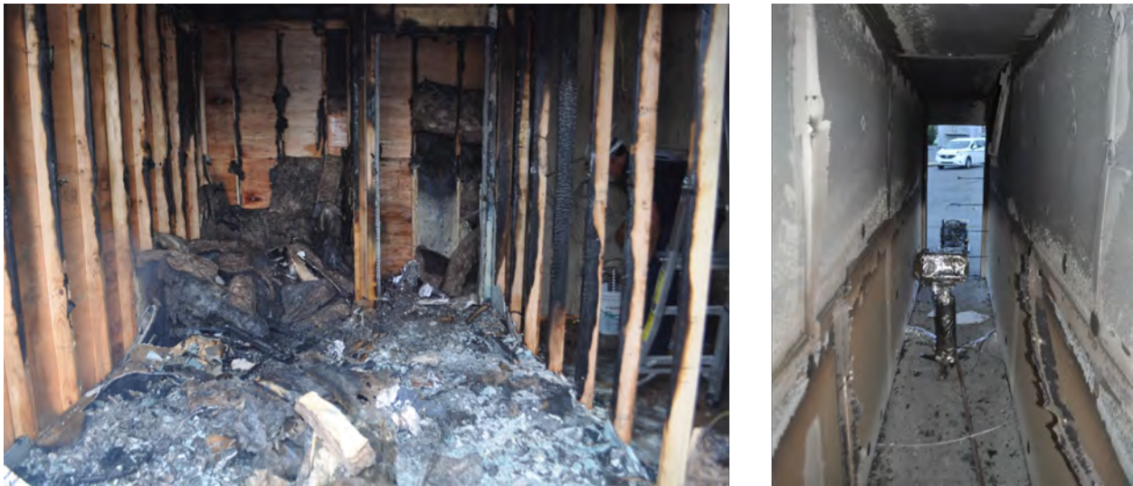
Figure 6.12: Images of the damage in the fire room (left) and hallway (right) of the Gypsum Prop after a single training fire with the pallets fuel load. The damage was caused by the fire and overhaul operations conducted to completely suppress the fire. After every fire, the gypsum board lining the inside needed to be replaced.
