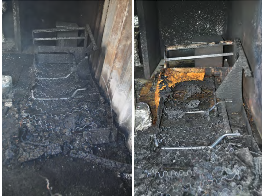
Figure 5.16: Images of the furniture fuel package after suppression from the tests with the vent door (left) and vent window (right) configurations. More fuel (end of the couch, carpet and padding near doorway, etc.) remained after the test with the vent window configuration than after the test with the vent door configuration.
