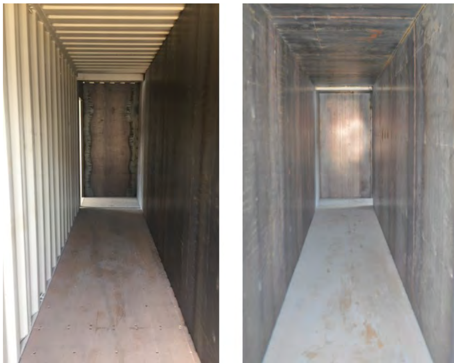
Figure 3.5: Images of interior wall linings of the Metal Prop (left) and Insulated Metal Prop (right). Both views are looking down the hallway towards the fire room.
