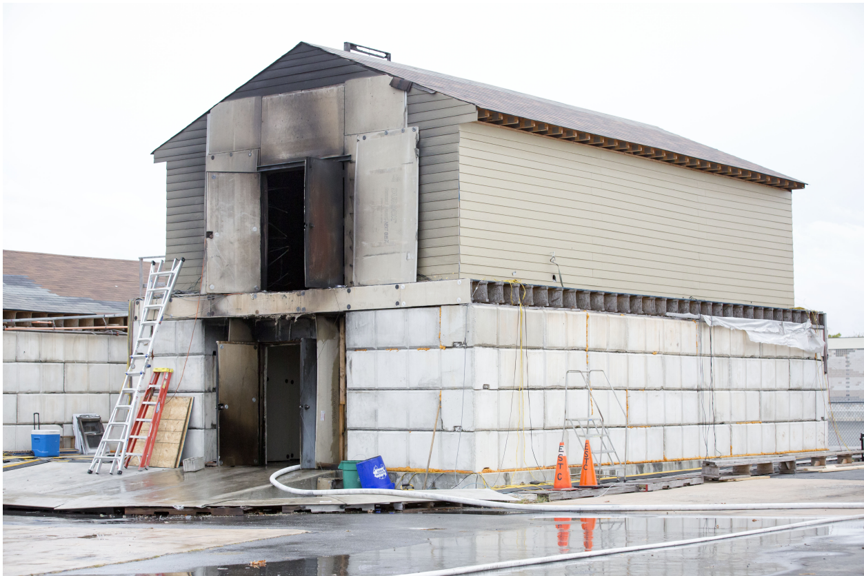
Figure 3.1: Delaware County, PA Fire Test Structure
