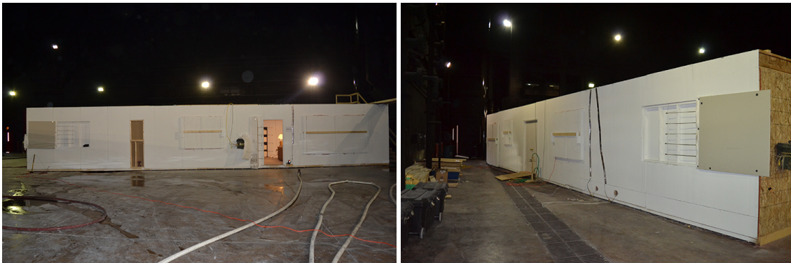
Figure 4.1: Exterior photos of test structure in UL's large fire lab. Side 'A' (left) and Side 'C' (right).
