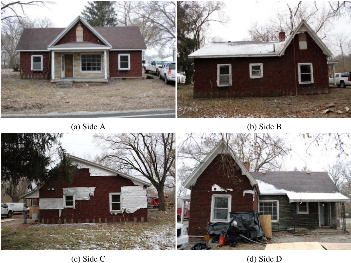
Figure 3.187: Exterior photographs of the structure for Experiment 16.
