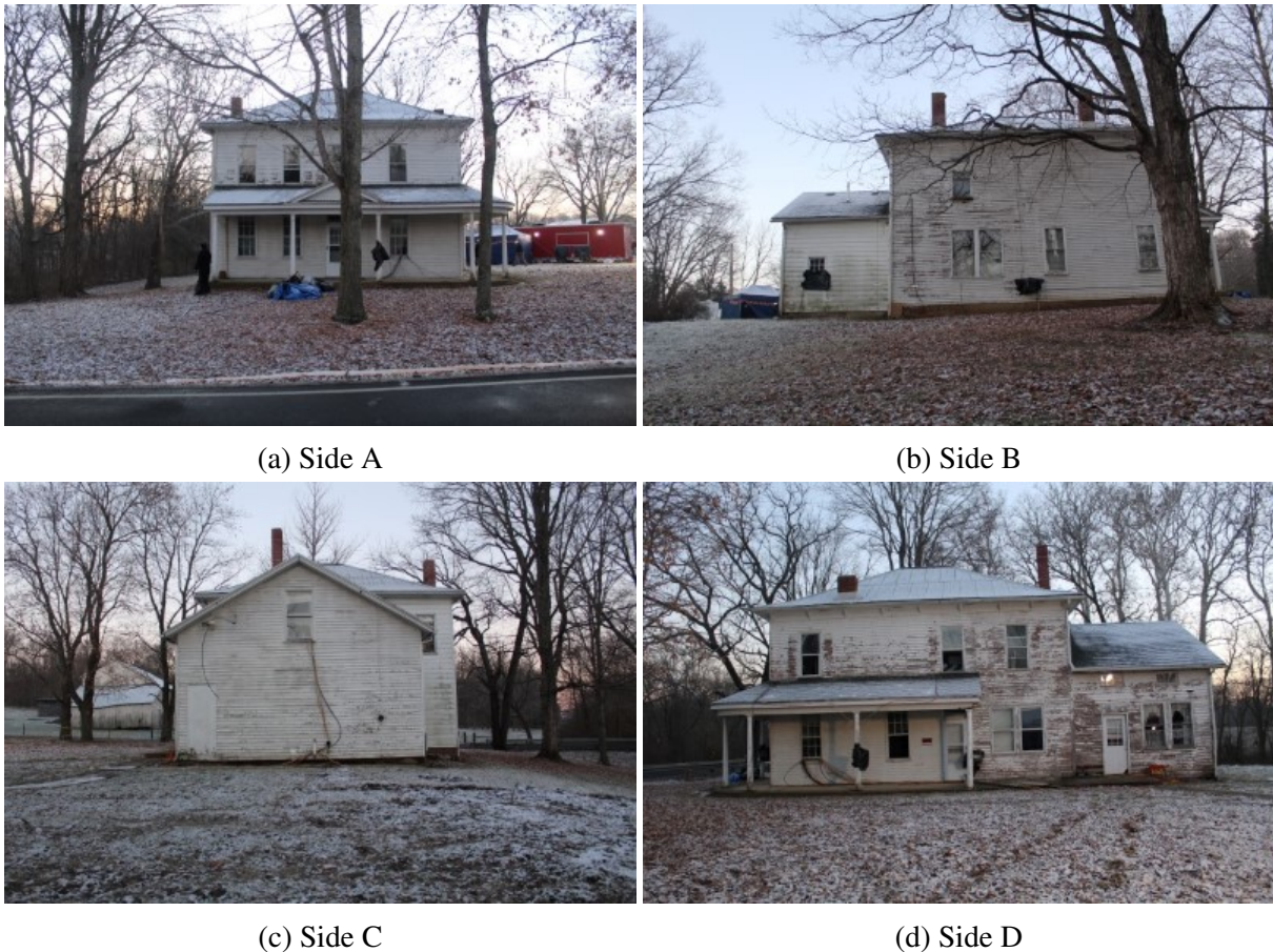
Figure 3.61: Exterior photographs of the structure for Experiment 6.
