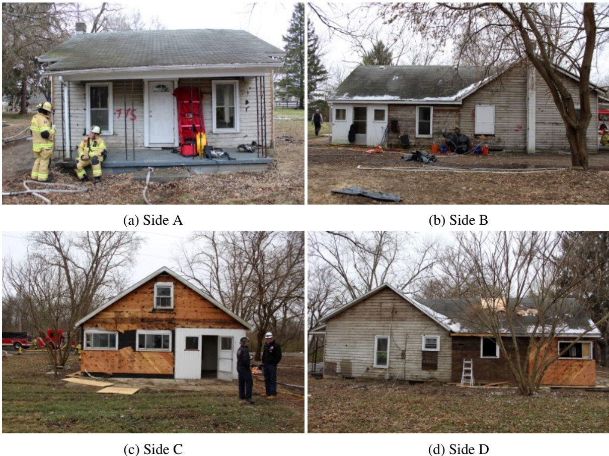
Figure 3.174: Exterior photographs of the structure for Experiment 15.
