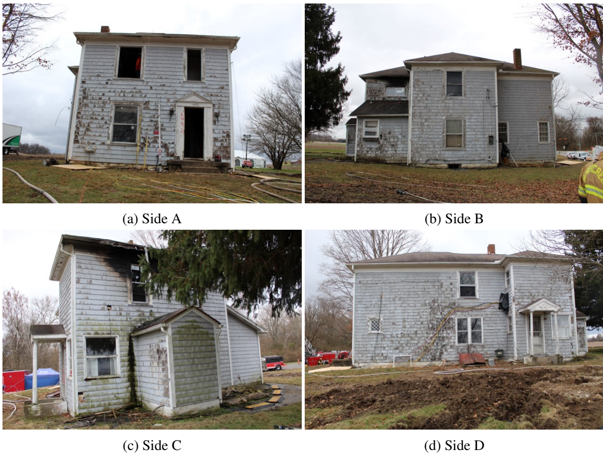
Figure 3.26: Exterior photographs of the structure for Experiment 3.
