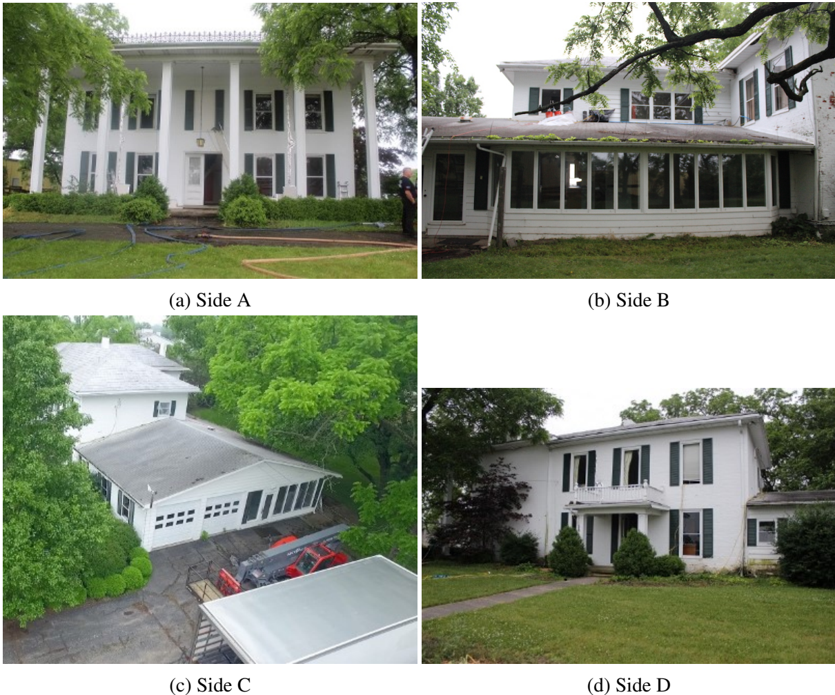
Figure 3.39: Exterior photographs of the structure for Experiment 4.
