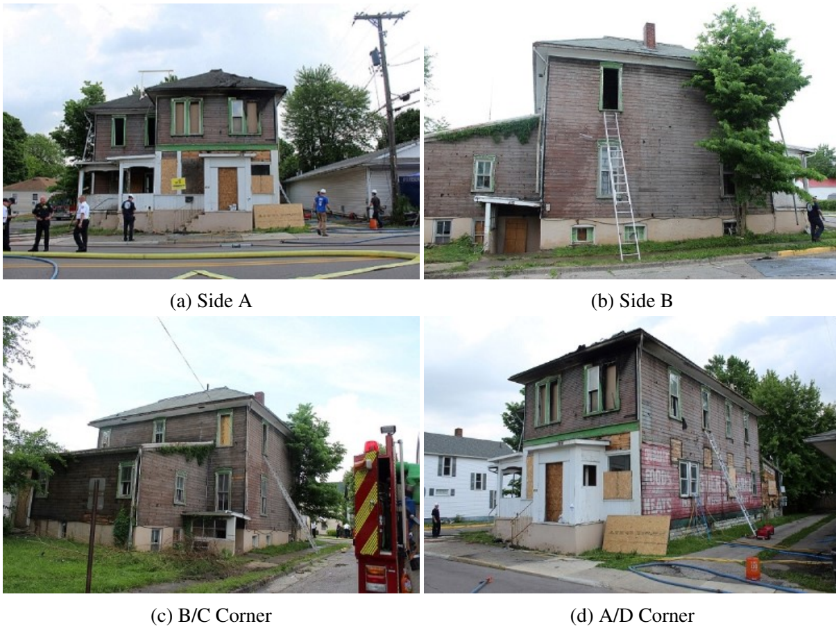
Figure 3.86: Exterior photographs of the structure for Experiment 8.
