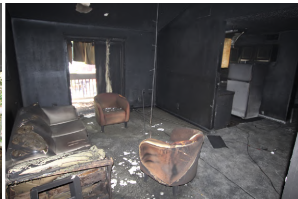
(b) Apartment F (Non-Isolated) Post Fire
