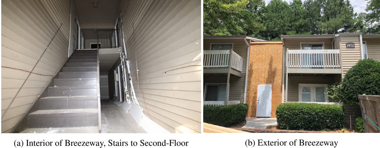
Figure 2.5: Exterior and interior views of the apartment breezeway, including the constructed wall to enclose the space.
