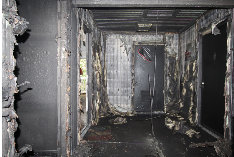
Figure 5.16: Post fire conditions as seen from the second-floor landing in Experiment 5. Note the extreme damage to the area with a limited view into Apartment H, which was isolated early into the experiment, maintaining survivable space.
