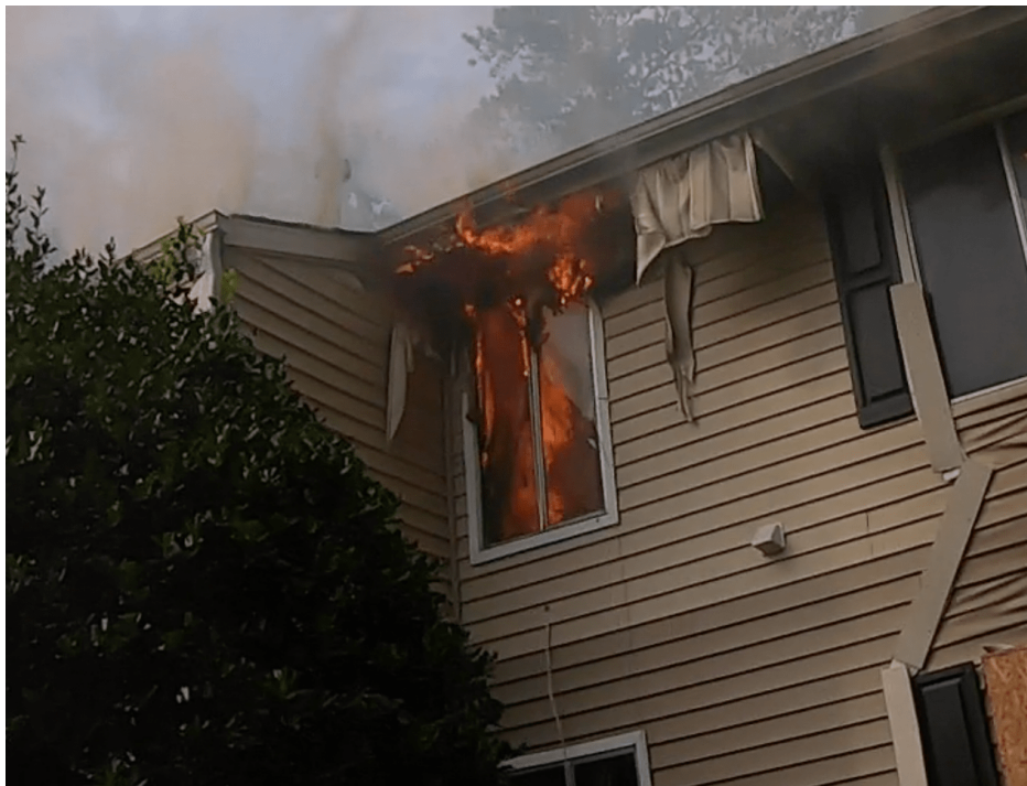
Figure 3.125: An image showing the degree of damage to the kitchen window by 707 s (11:47) post ignition (73 s prior to firefighter intervention) in Experiment 4A.
